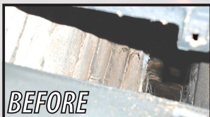
Exposed Brick Corbells Before HeatShield Cerfractory Foam
