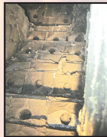
Jagged Corbelling and Exposed Brick Cores (Holes) in a Smoke Chamber
