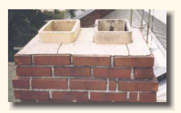
A chimney crown is the masonry covering at the top of your chimney. Its purpose is to prevent water from seeping through to the chimney below. When the crown fails, the entire chimney system is susceptible to damage.
