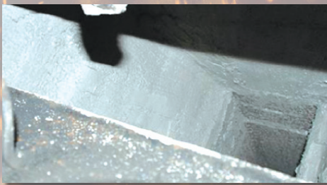
Streamlined smoke chamber wall after HeatShield Cerfractory Foam
